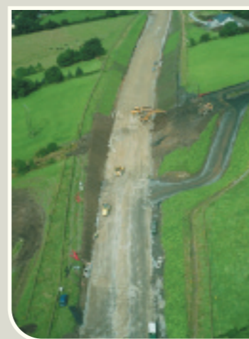
Aerial view of scheme under construction.
